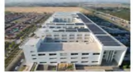
PMGD Cintac, Maipú, 2.88 MWp
