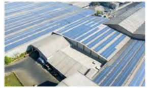
Net-Billing CESFAM San Clemente, 35 kWp
